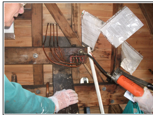
Using a grease gun for the fantail bearings
